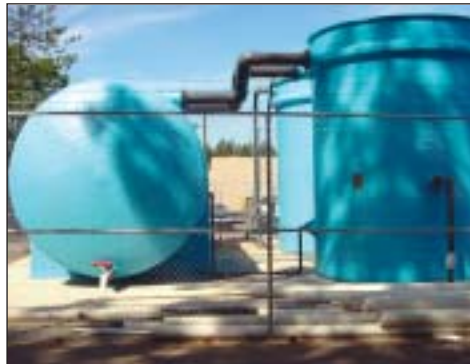
IWS installed the modified SBR as part of the new treatment system.
