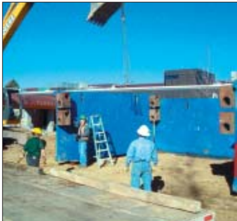
Box shoring was utilized to assure a safe work environment
