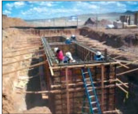
60,000 gal cast in place concrete tank formed by IWS crew.
