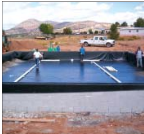
Constructing 10,000 GPD lined sand filter.
