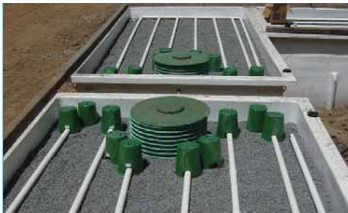
Living Machine® in process of construction
