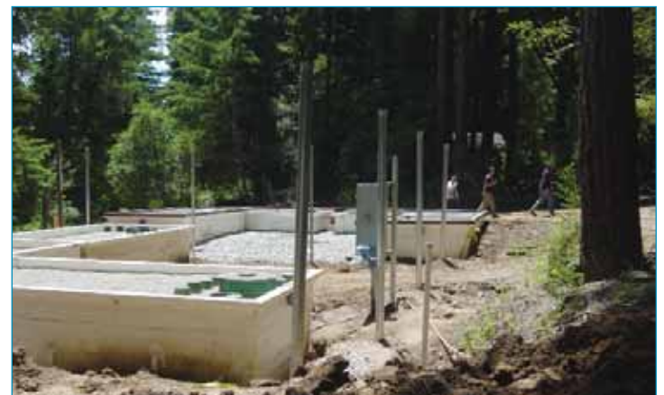
Layout of Living Machine® cells at site
