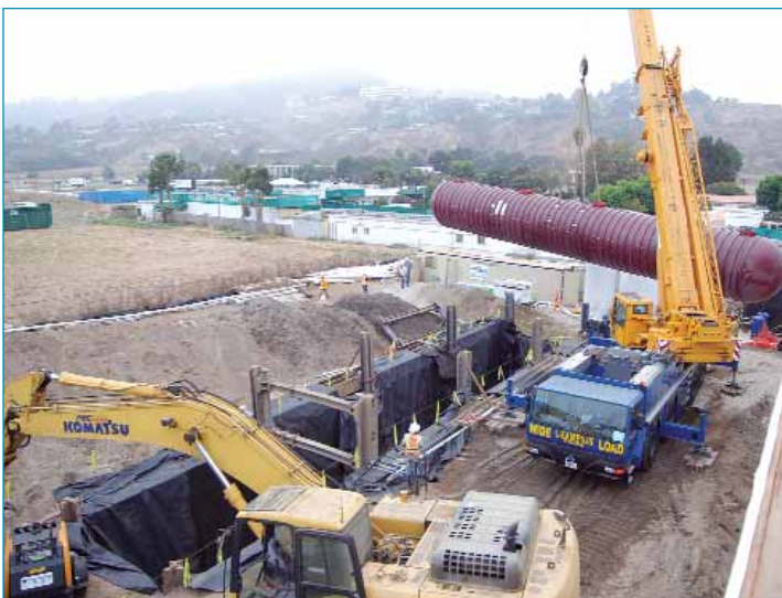
Installation of 75 foot MBR Treatment Tank through shoring structure
