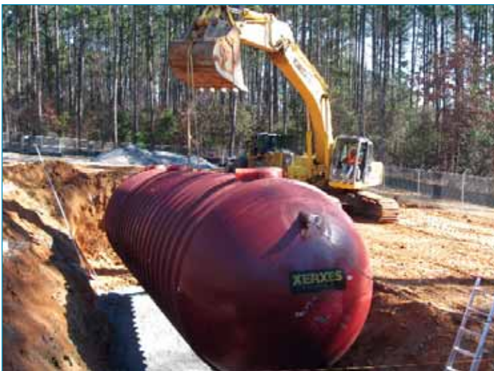
Setting tank a 30,000 gallon septic tank
