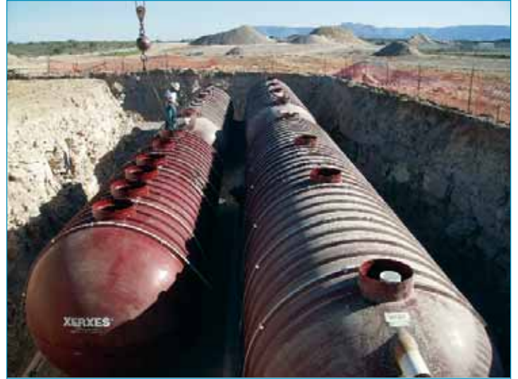
Tanks set in excavated bedrock
