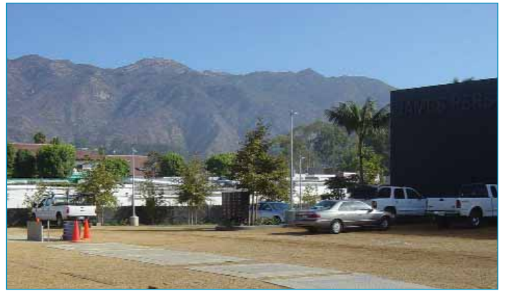
Covers on MBR vaults in the parking lot
