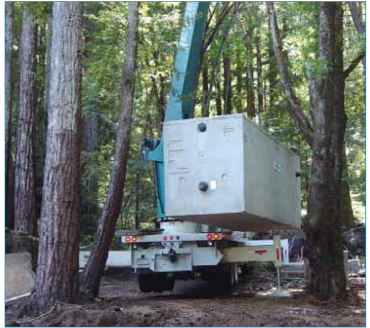
Setting Jensen Precast Tank in wooded area
