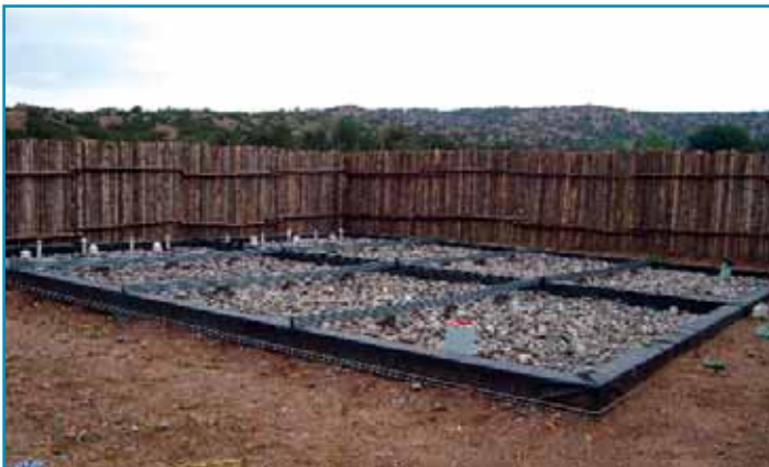
IWS Upflow Filter enclosed in coyote fence
