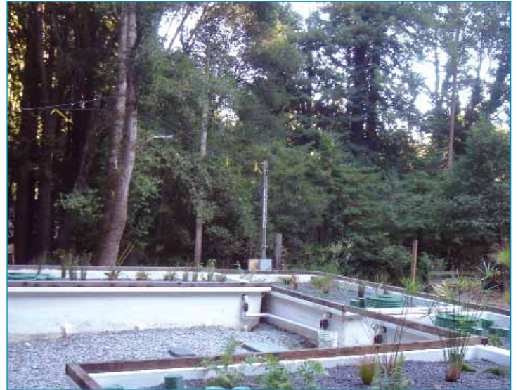
Living Machine® System treatment cells
