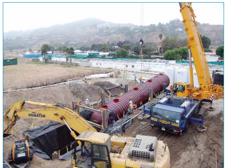
Installation of 75 foot MBR Treatment Tank through shoring structure
