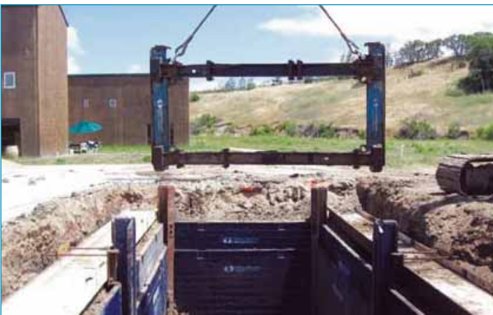
Installing slide rail shoring prior to setting the tank
