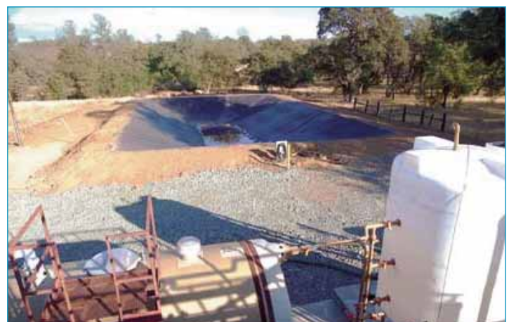
View of construction holding pond
