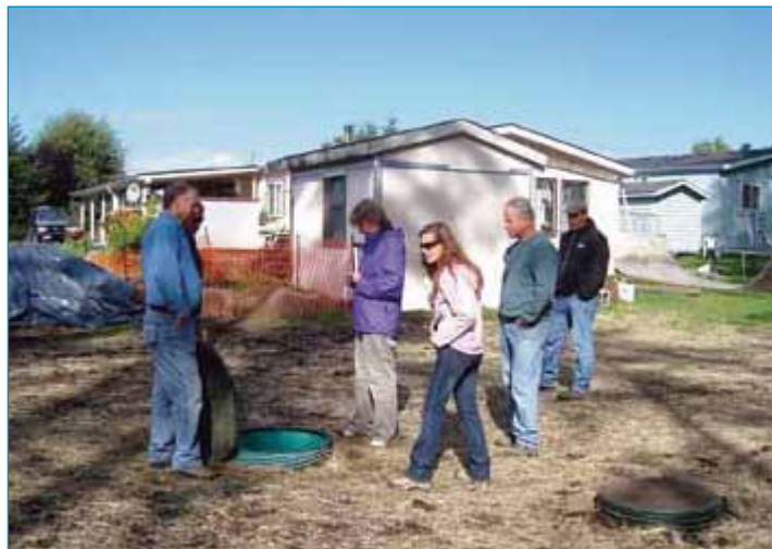
Project involved work in close proximity to homes
