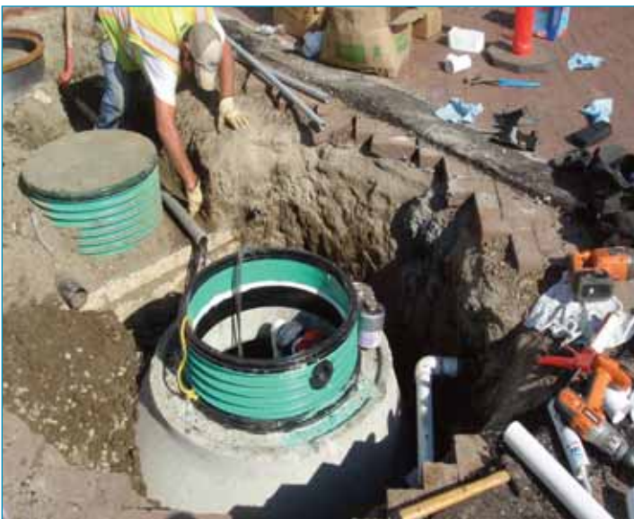
Replacing a pump vault manhole access cover
