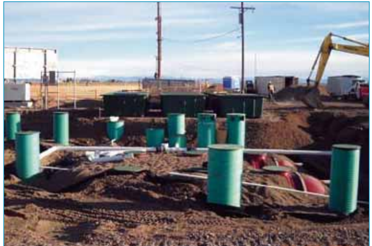
Treatment system being installed
