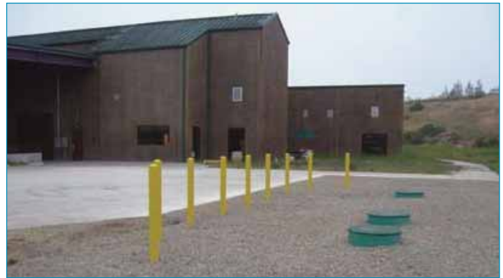
The completed tank installation adjacent to the concrete pad
