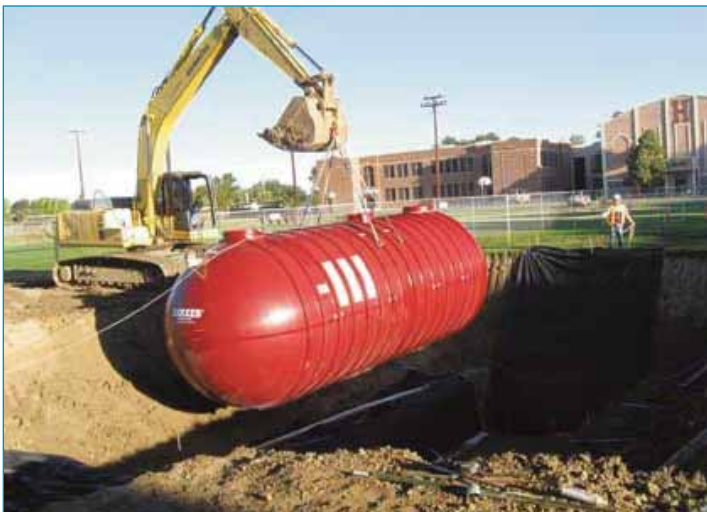
Setting the Xerxes Tank
