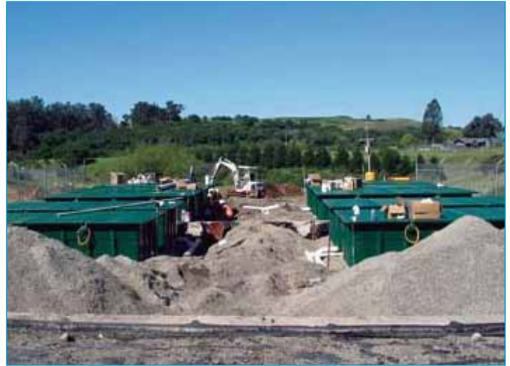
Advantex system under construction
