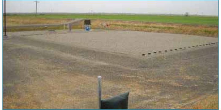
Recirculating Sand Filter
