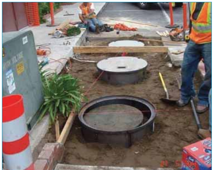
Completing repair of tank and pump vault risers in planter area
