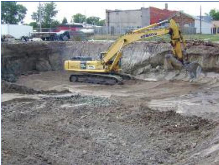
*Contaminated soil is excavated and removed from the project site*
