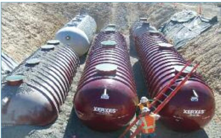
*The two ENR Denite units are set in the foreground in the Xerxes tanks*
