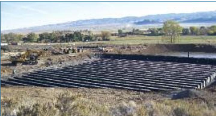
An at grade and elevated view of the Infiltration Basin field
