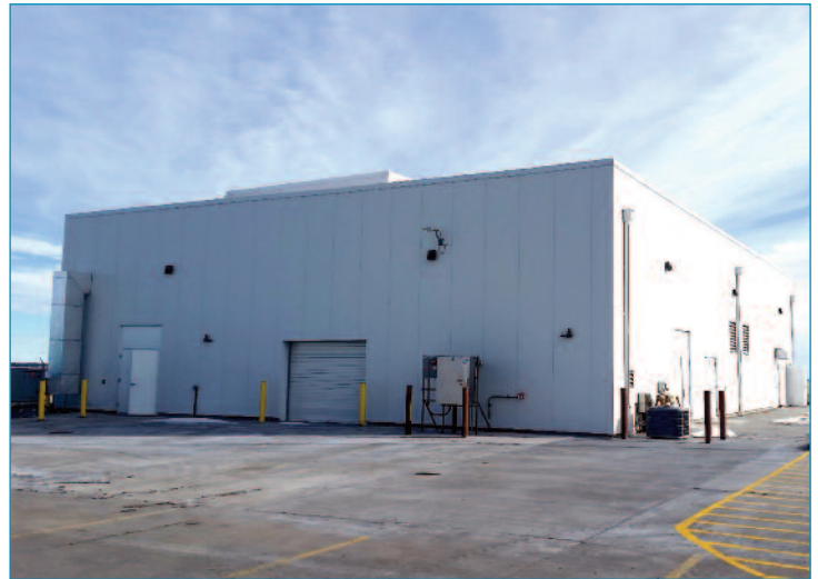
Completed Treatment Building
