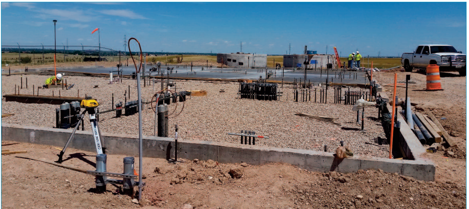
Building foundation with penetrations
