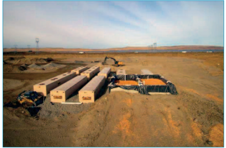
Wastewater Treatment System During Installation
