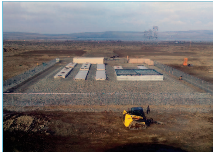
Wastewater Treatment System After Final Grading
