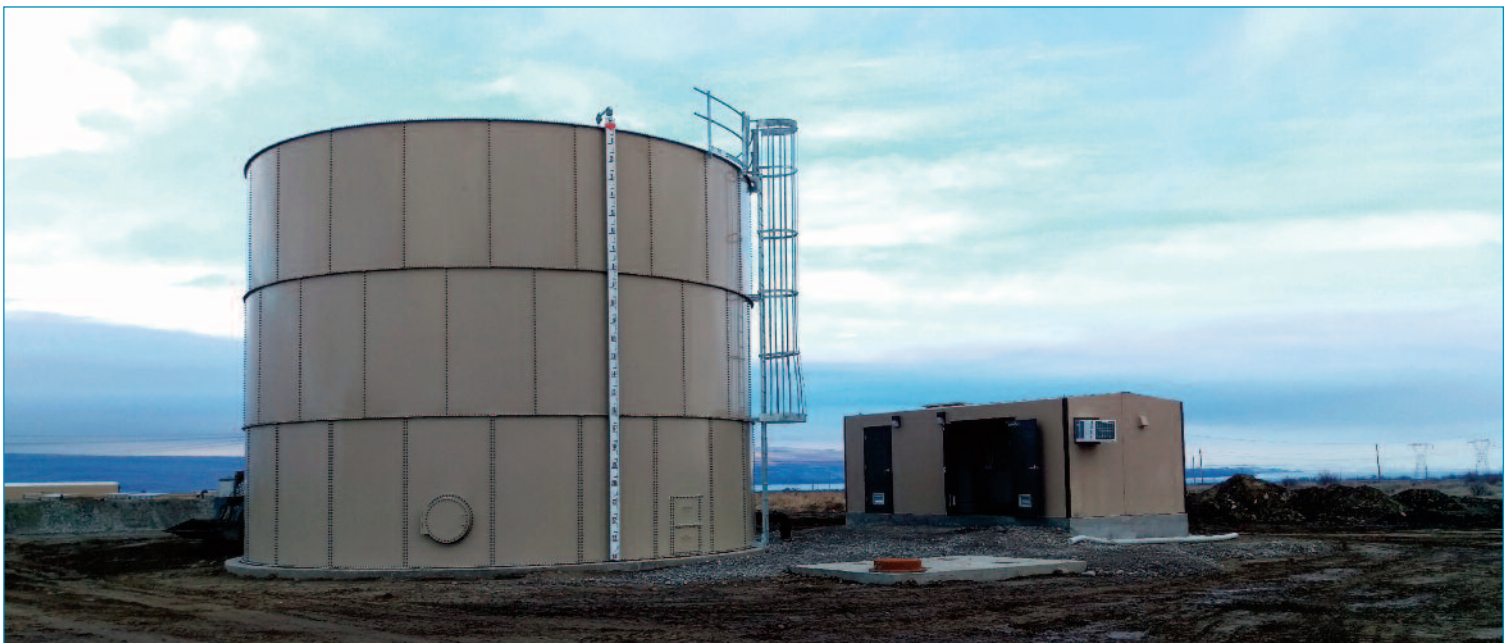
Water Treatment System
