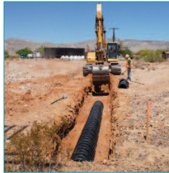
Installing the infiltrator chambers
