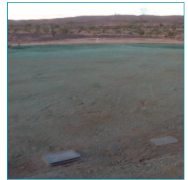
Final view of the leachfield
