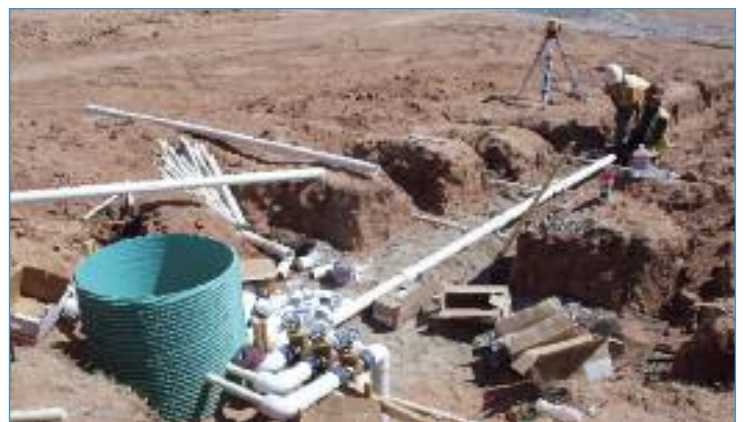
Installing the LPD field piping
