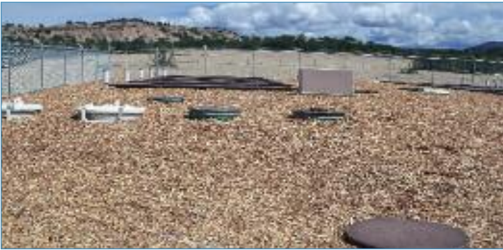
The completed treatment system installation
