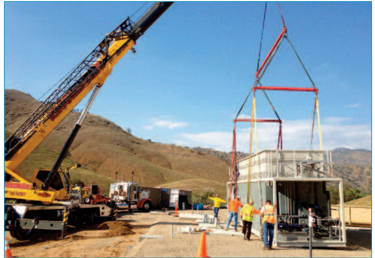
Off loading microBLOX unit
