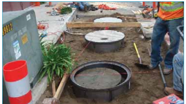
Completing repair of tank and pump vault risers in planter area
