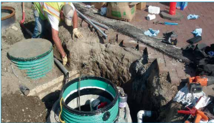
Replacing a pump vault manhole access cover
