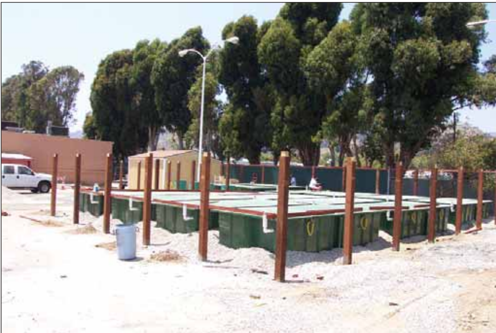
Orenco Advantex Treatment Pods prior to fence installation
