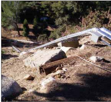
Steep grade and environmental conditions required insulated pipe and special design features
