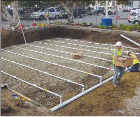
Drainfield installation in parking lot area
