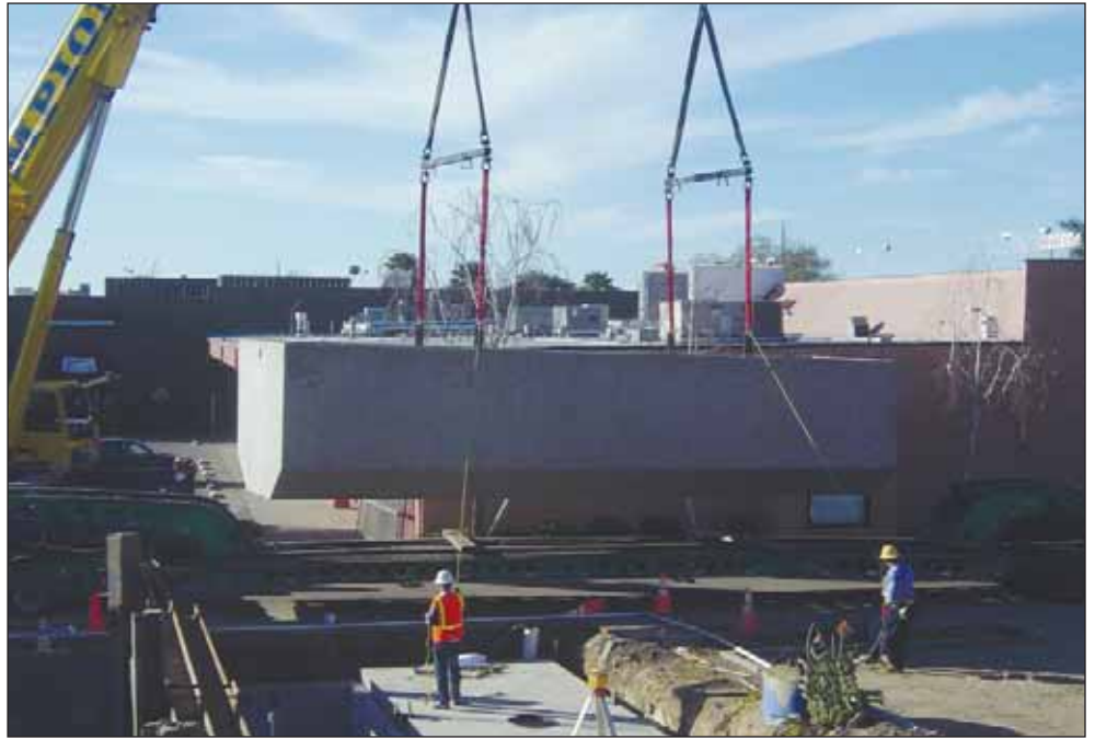
Large concrete tanks required special transport and handling
