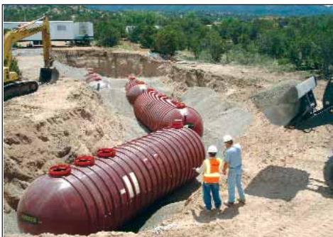
Installation of four 20,000 Gallon Tanks (Primary and Recirc)
