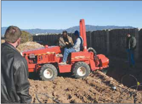
IWS preparing to install drip irrigation with vibratory plow
