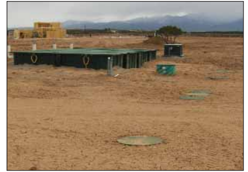
Construction of treatment system nears completion
