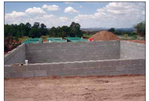
Construction of the outer perimeter of the Upflow Nitrogen Reduction Filter
