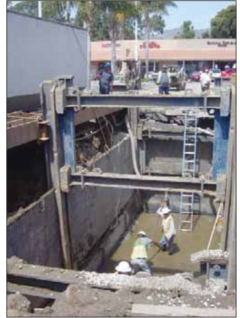
The Double Whammy – Box shoring and Dewatering required for tank installation
