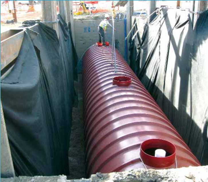
IWS setting tank in shored structure
