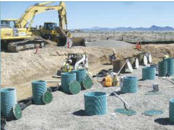
The tank area backfilled with risers installed
