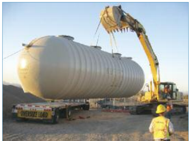
Off-loading the Septitech Treatment Vessel
