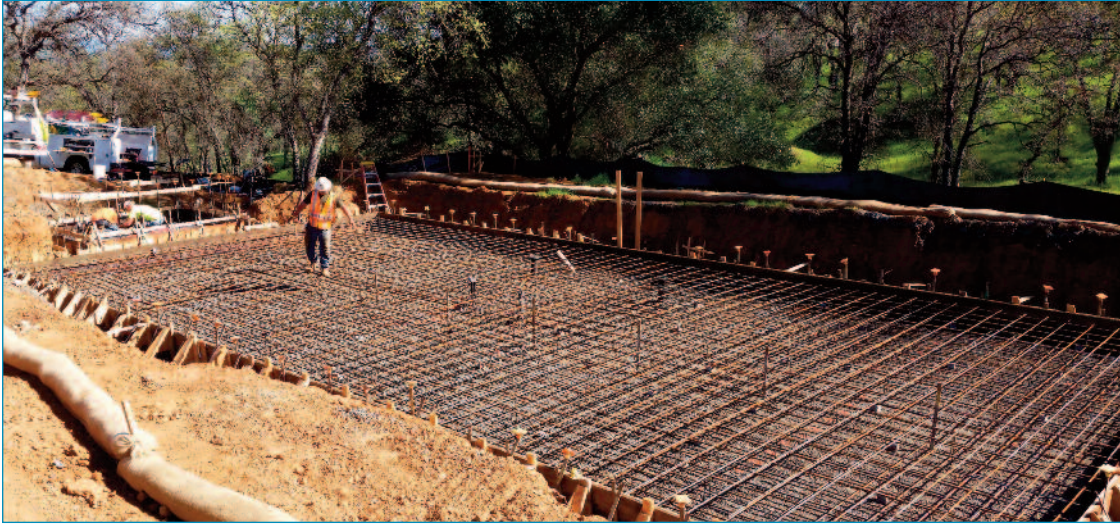
Rebar for Pad
