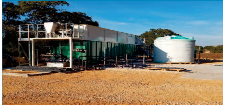
Constructing MBR System
