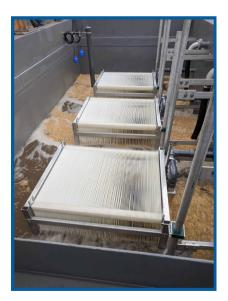
Membranes in immersed MBR systems are commonly configured in two ways: as hollow fibers grouped in bundles, or as flat sheets. Flat sheet products can be further divided into rigid plates and flexible flat sheet types. Other configurations and materials are available for niche applications such as multitube and ceramic products.
