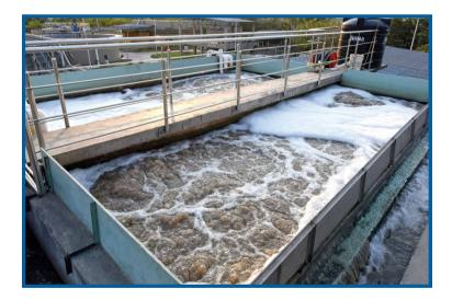
The cross-flow dynamic of the water against the membrane controls the buildup of material on the membrane surface. Air scouring is one way in which membranes in MBR applications are cleaner.
