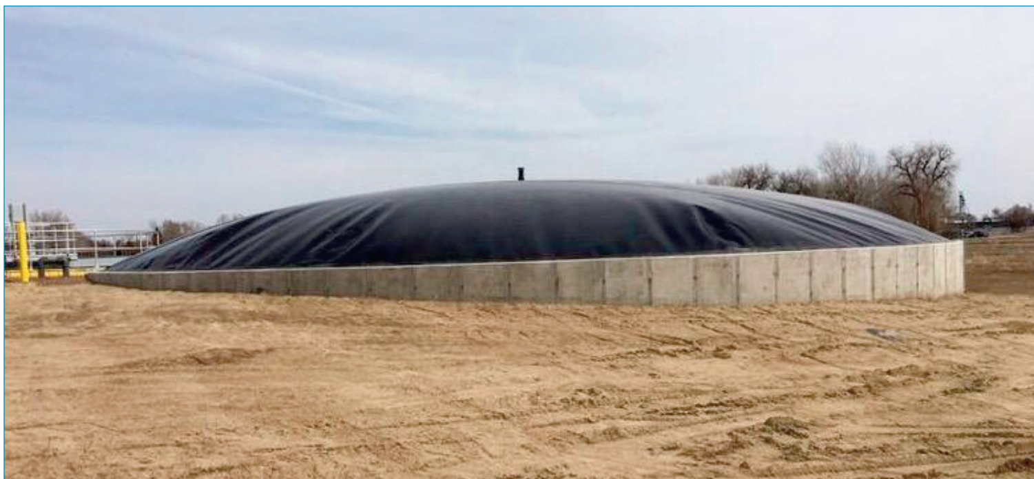
Newly Constructed Digester With Cover
