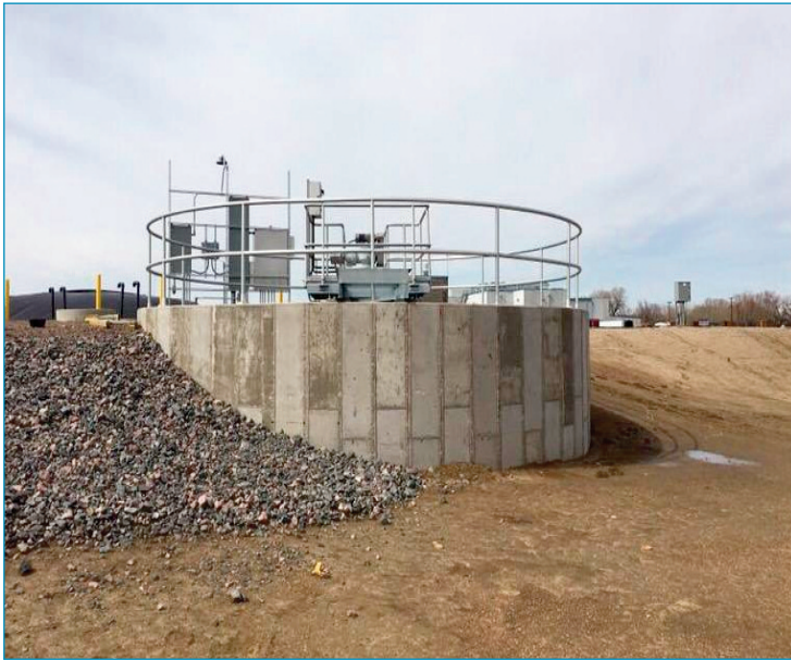
Newly Constructed Clarifier
