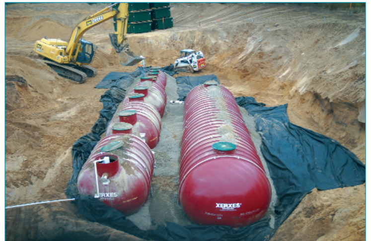
Tanks installed in excavation
