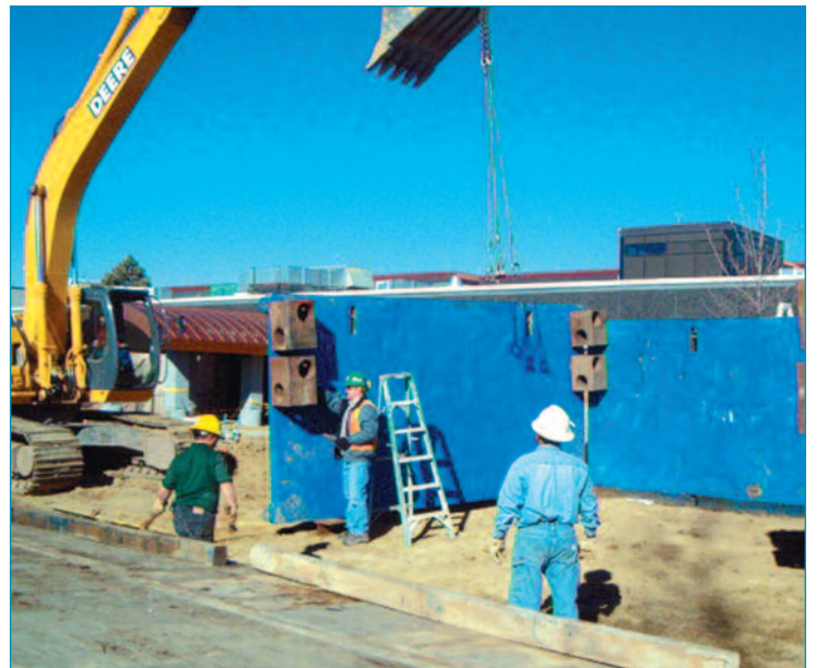
Box shoring was utilized to assure a safe work environment
