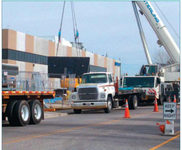
The project required coordinating multiple construction activities
