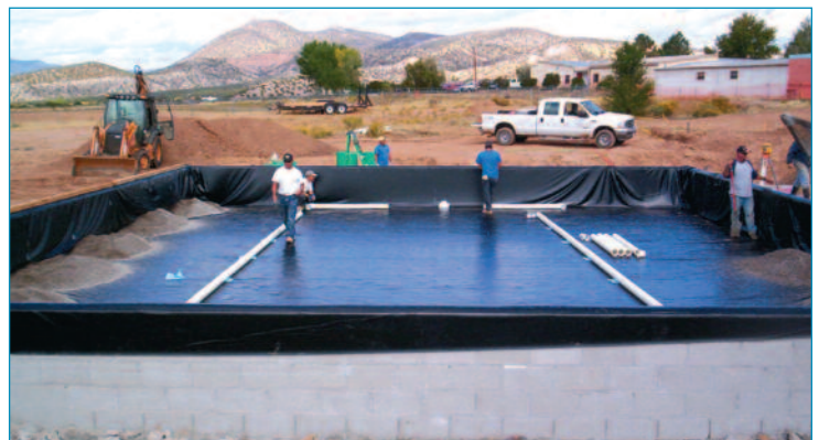
Constructing 10,000 GPD lined sand filter
