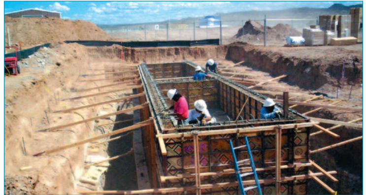
60,000 gal cast in place concrete tankformed by IWS crew
