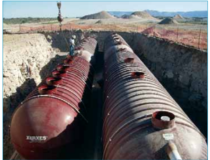
Tanks set in excavated bedrock
