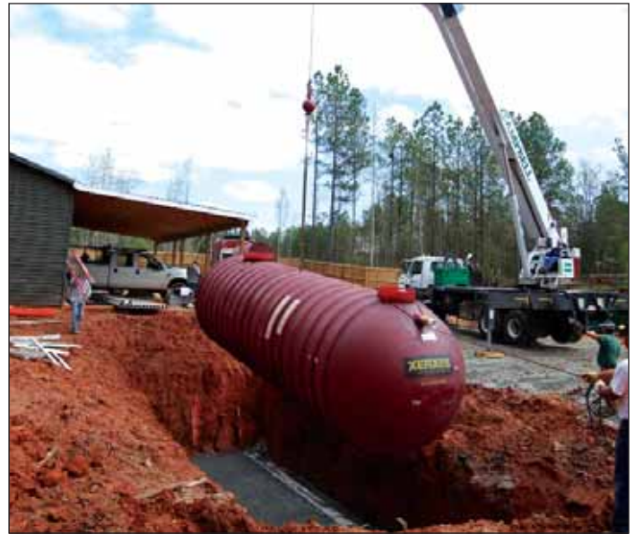
IWS setting Xerxes treatment tank
