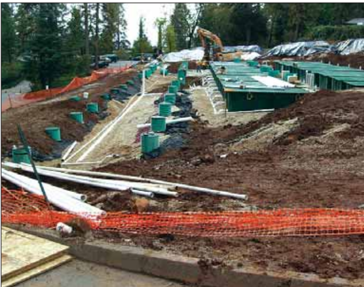
Treatment area being completed
