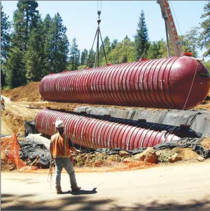
IWS setting large fiberglass tanks (40,000 gallon) in treatment area
