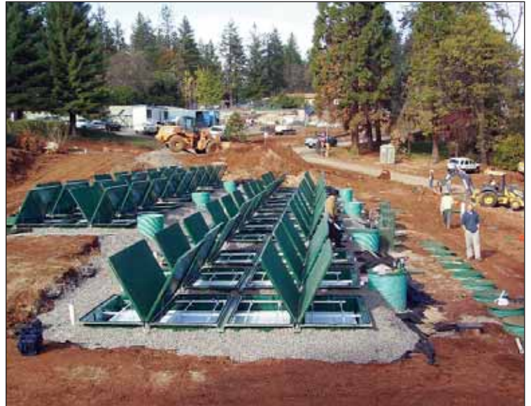
Orenco AX-100 pod open for inspection
