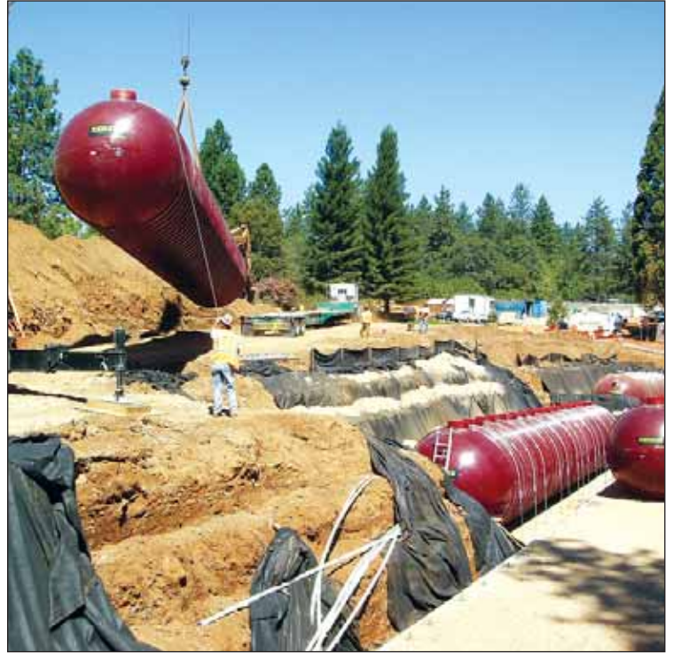
IWS setting large fiberglass tanks (40,000 gallon) in treatment area
