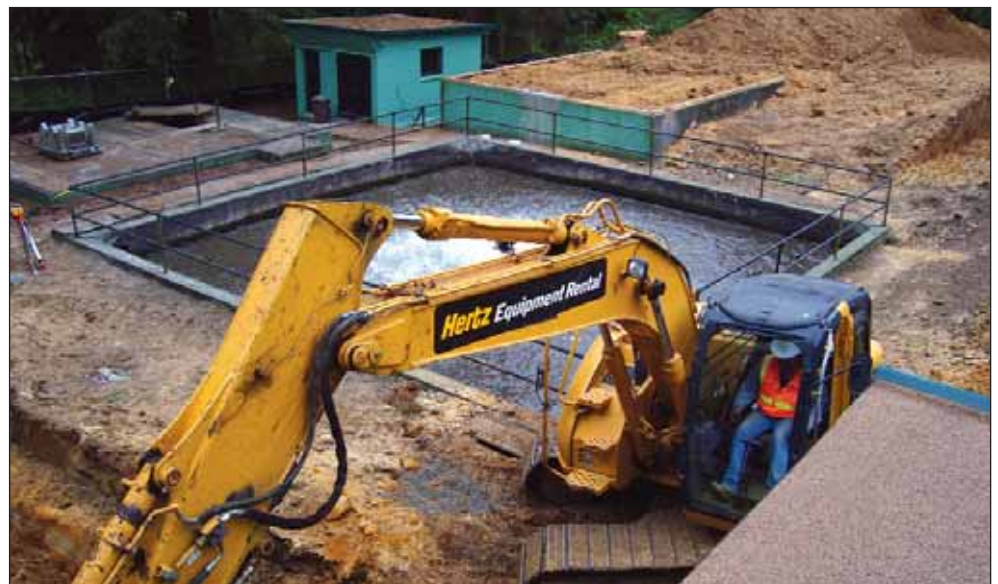
Installation of treatment system
