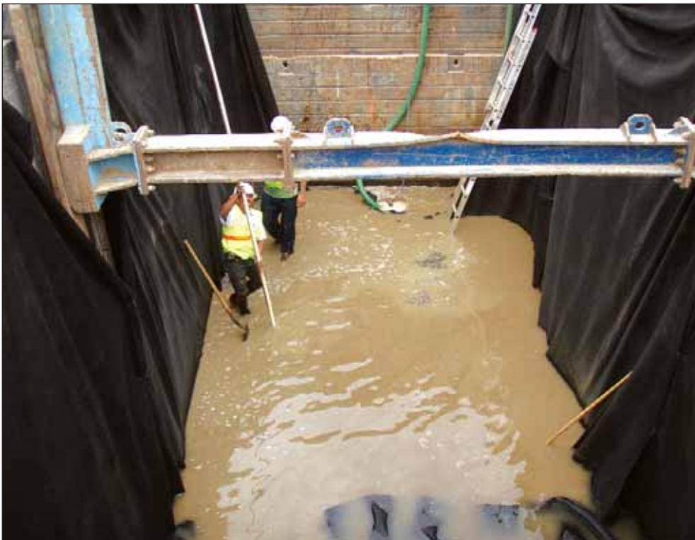
IWS shoring and dewatering of excavation to install tanks
