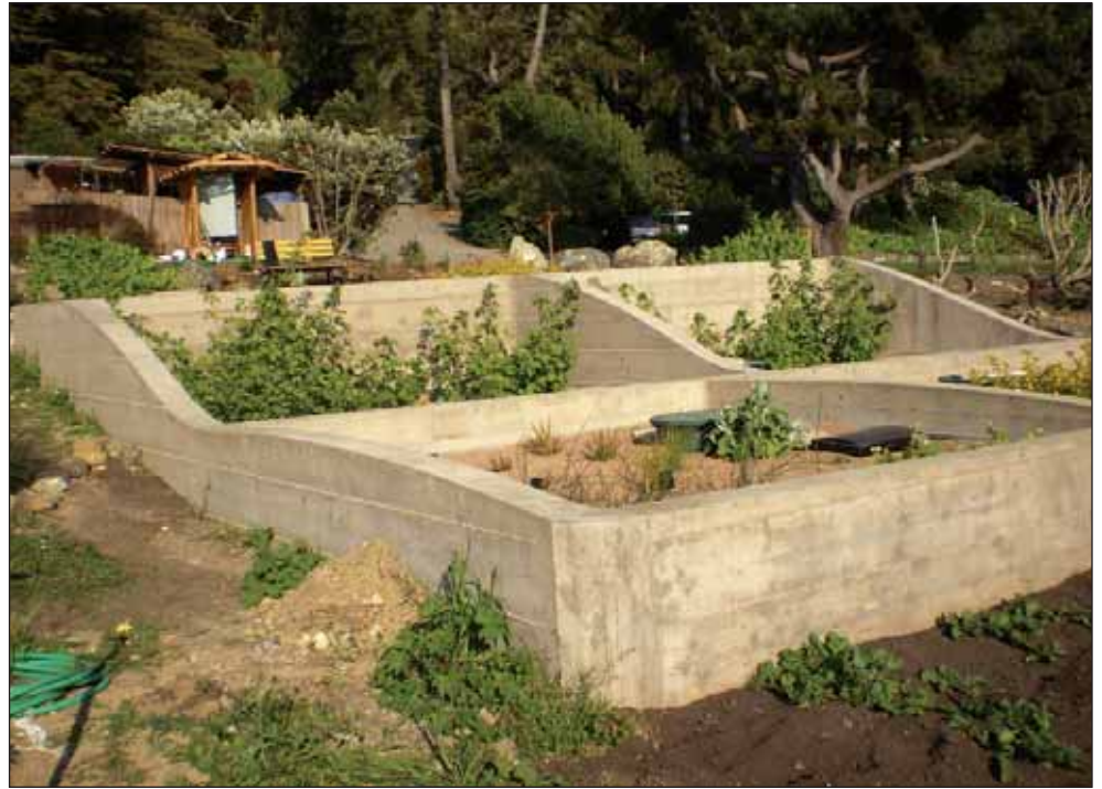
The Living Machine Concrete Wetland Cells
