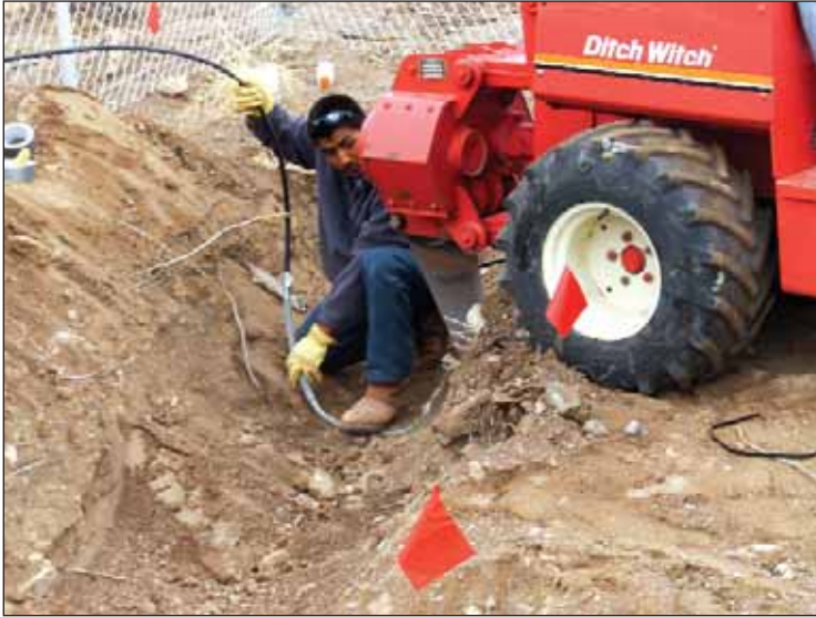
IWS preparing to install geoflow drip irrigation with vibratory plow
