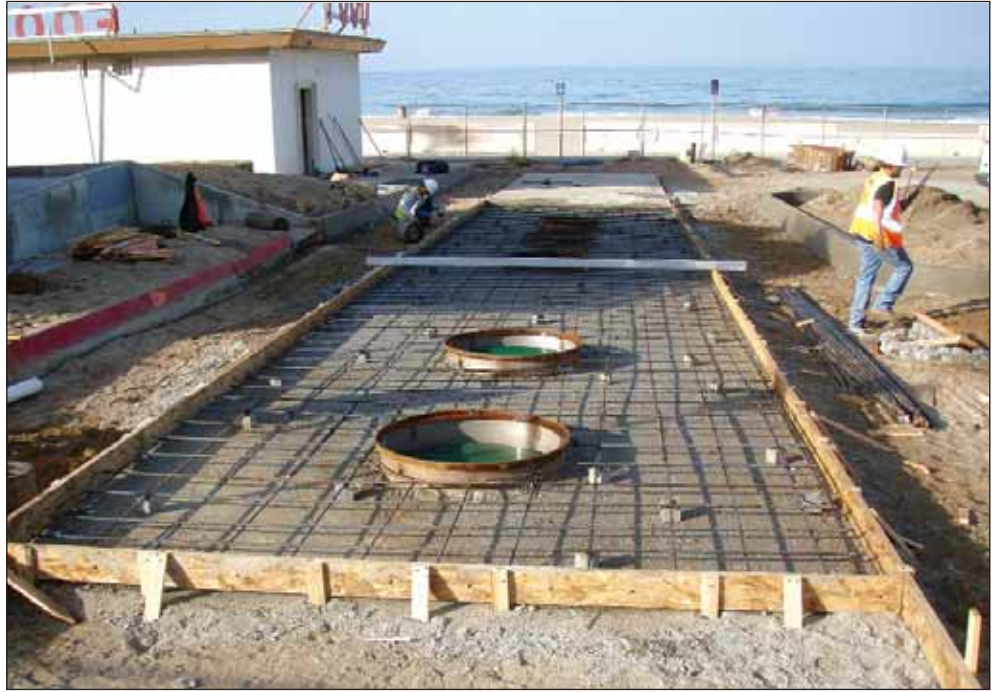
IWS installing forms for concrete covers on tanks
