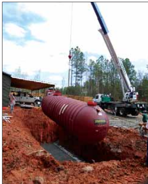
IWS setting Xerxes treatment tank
