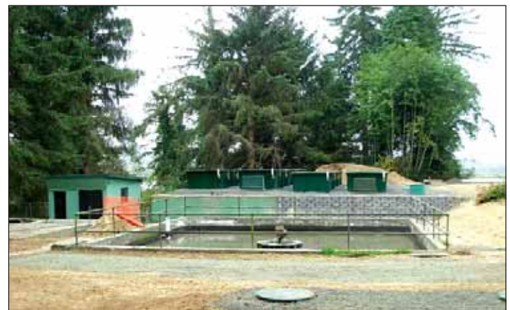
SSSD facility after upgrade was completed
