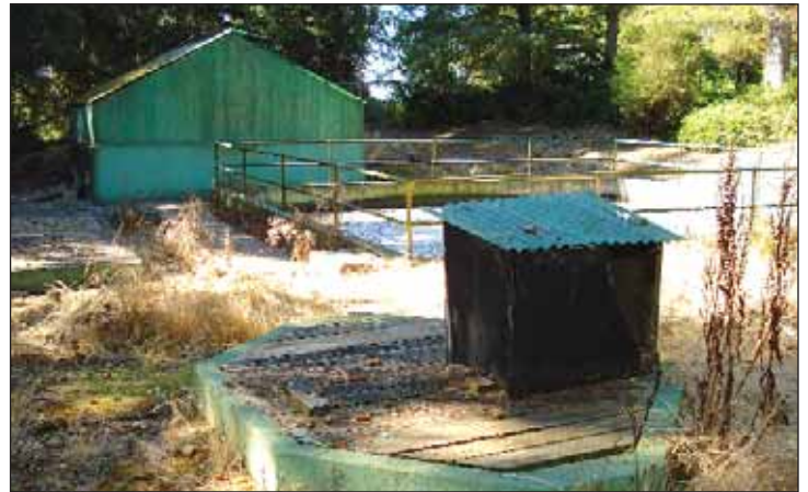
SSSD facility prior to upgrade
