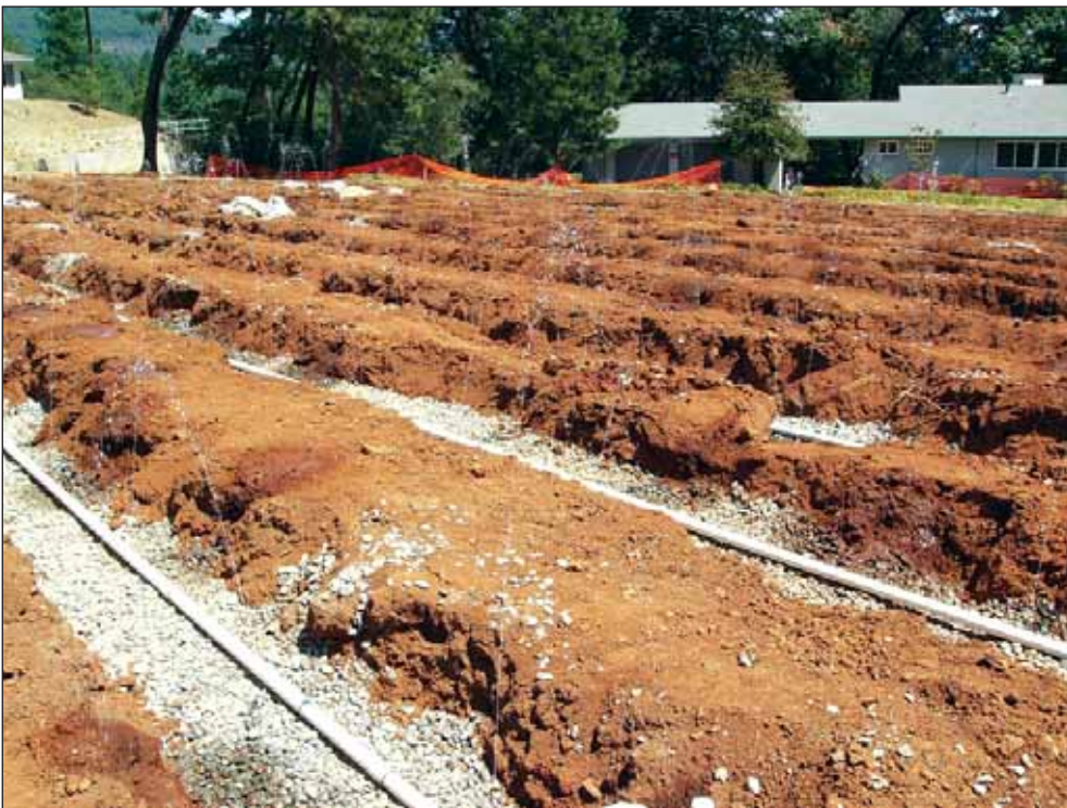
New drainfield undergoing squirt test
