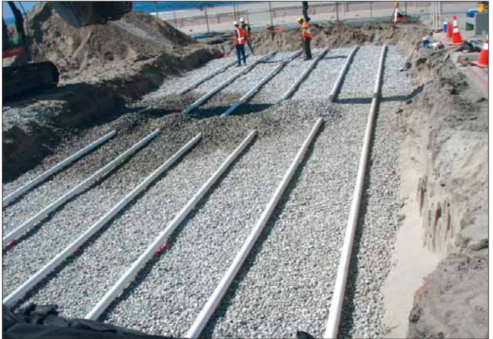
IWS drainfield installation at Zuma Beach
