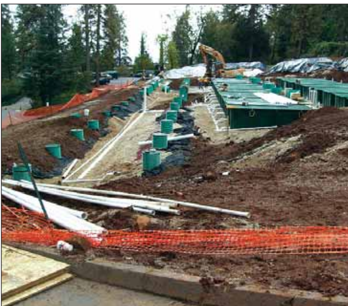
Treatment area being completed
