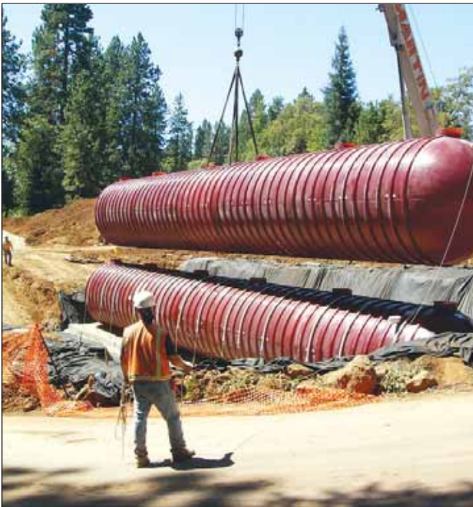
IWS setting large fiberglass tanks (40,000 gallon) in treatment area
