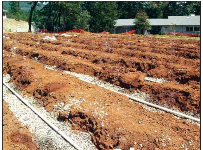
New drainfield undergoing squirt test
