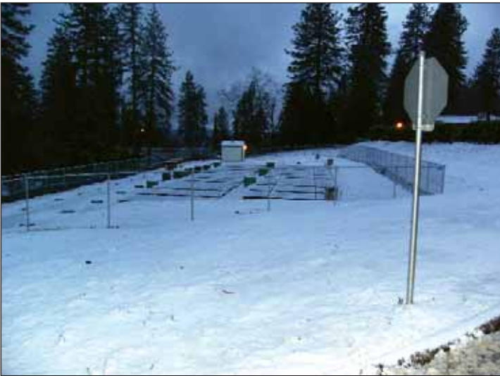
The completed treatment system after a dusting of snow
