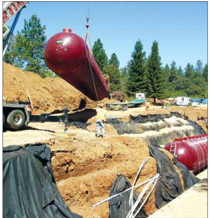
IWS setting large fiberglass tanks (40,000 gallon) in treatment area
