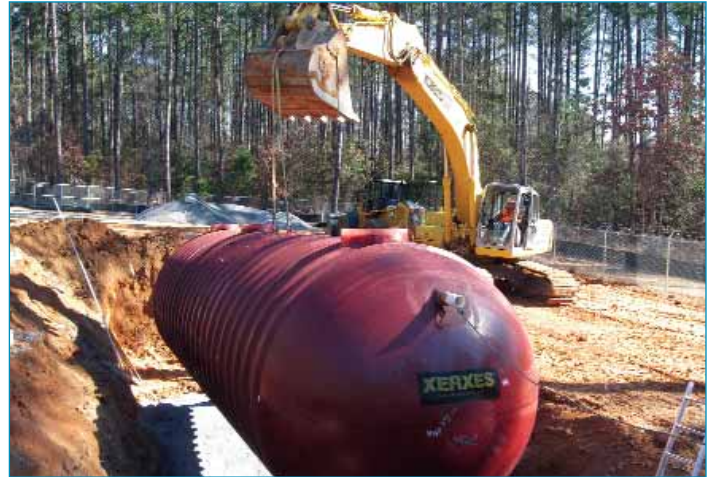
Setting tank a 30,000 gallon septic tank
