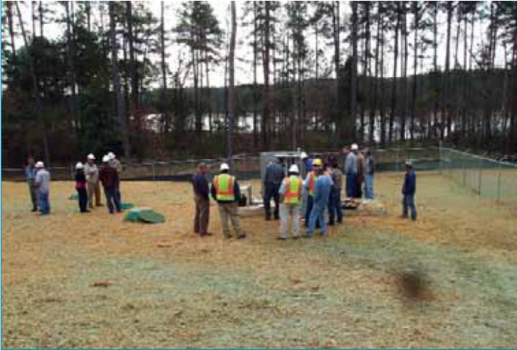
Project stakeholders and IWS at the system start-up
