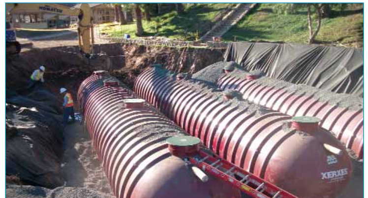
Large fiberglass tanks being installed
