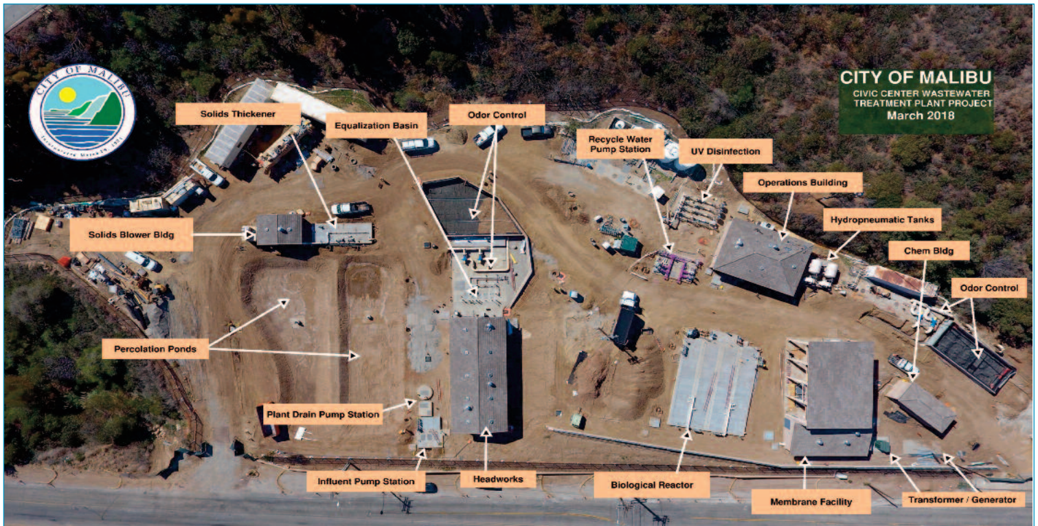
Treatment Plant Components
