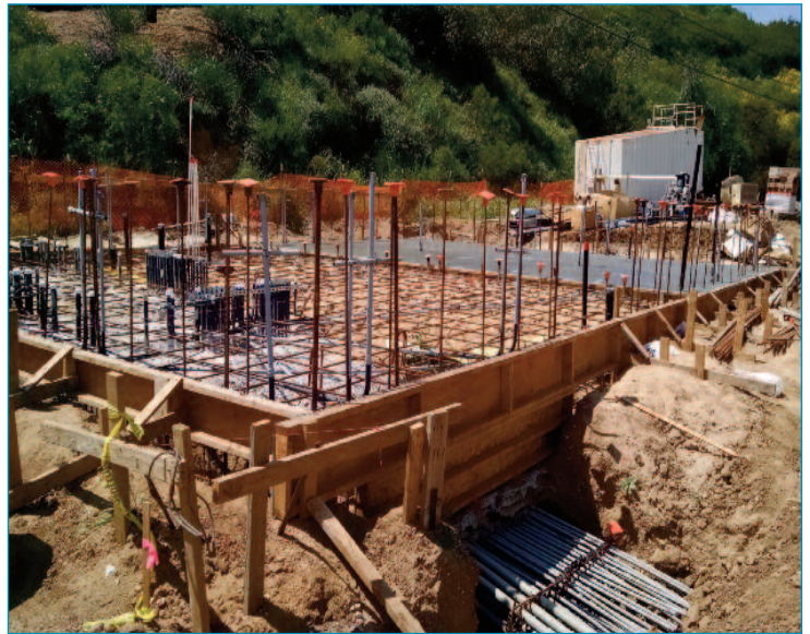
Conduit penetrations and stub outs for the control building
