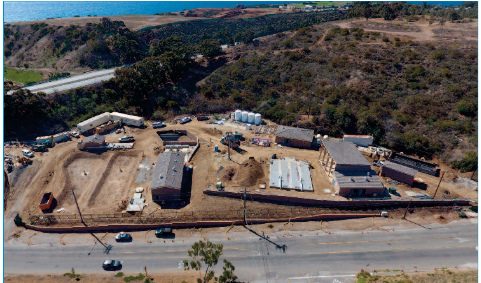
Treatment Plant Overview
