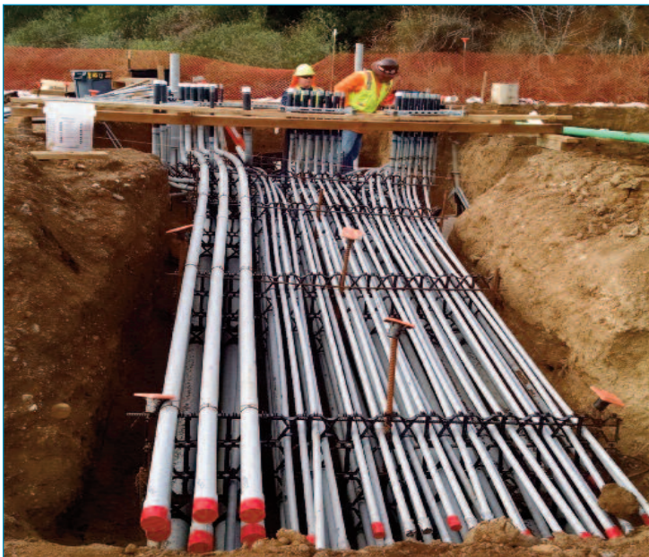
Duct Bank to MBR Building
