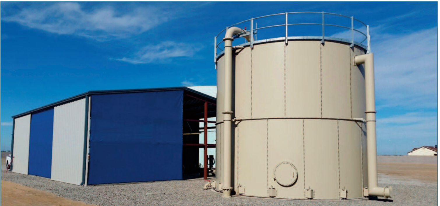
Treatment Building and Reclaim Storage Tank
