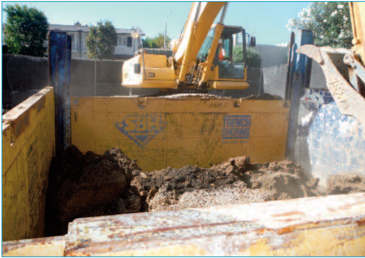
Shoring to protect nearby structures
