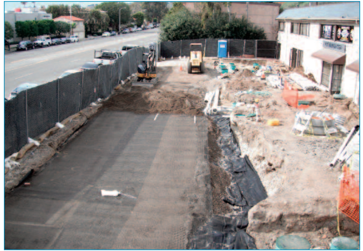
North parking lot drainfield completed
