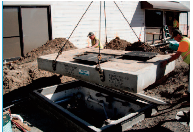
Installing lid on precast concrete tank
