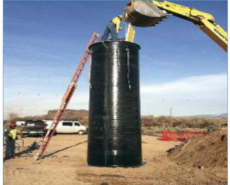
Preparing to set packaged lift station
