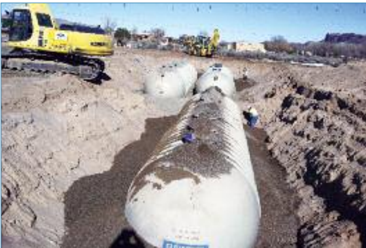
Containment Solutions treatment tanks
