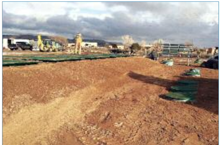
Advantex treatment pods and tank risers after backfilling
