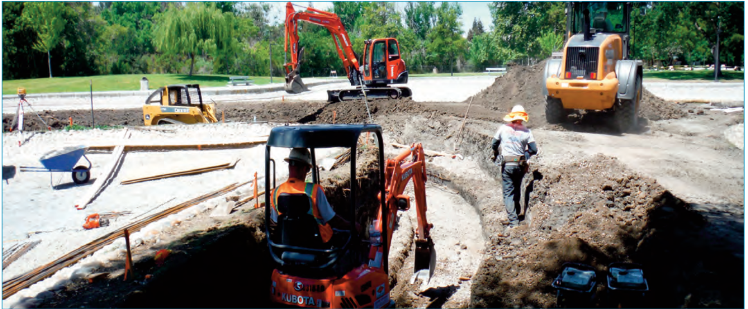
Site work in constructed wetlands treatment area
