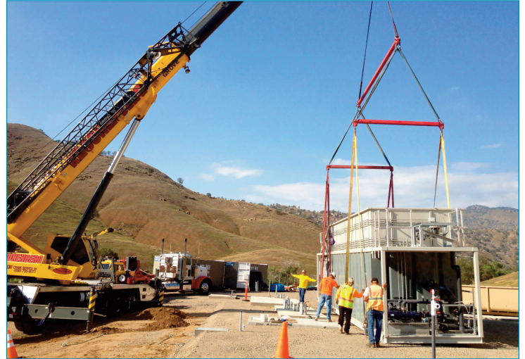
Off loading microBLOX unit
