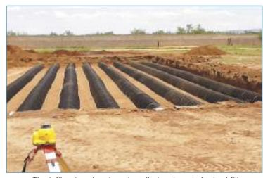
The infiltration chambers installed and ready for backfill
