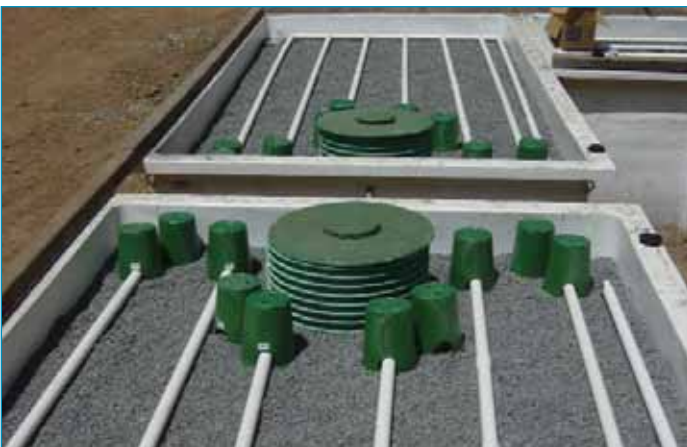
Living Machine® in process of construction
