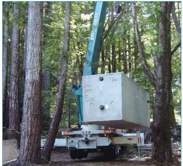
Setting Jensen Precast Tank in wooded area
