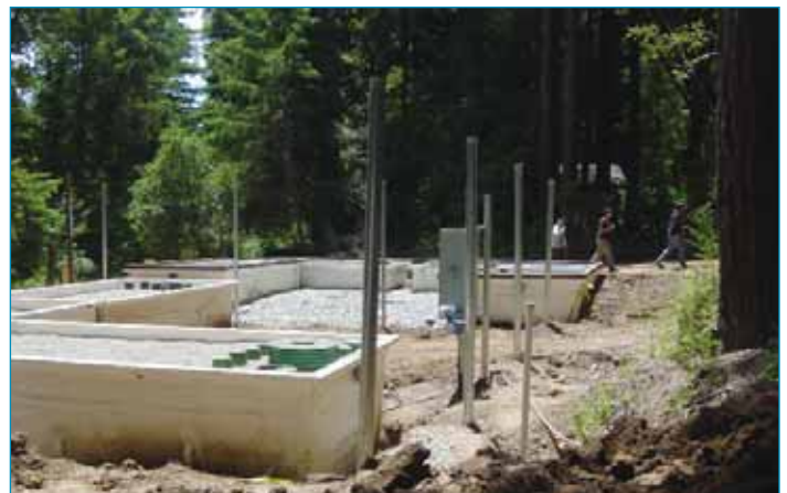
Layout of Living Machine® cells at site
