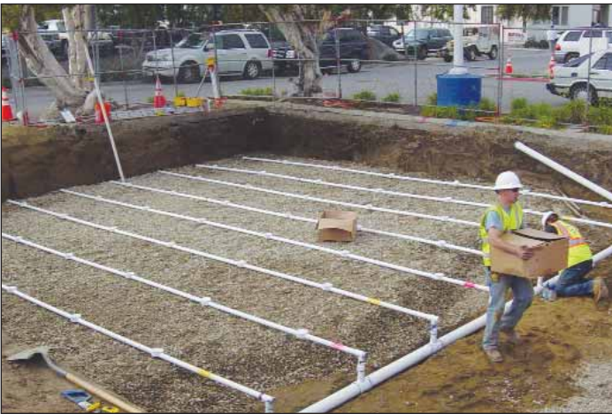
Drainfield installation in parking lot area
