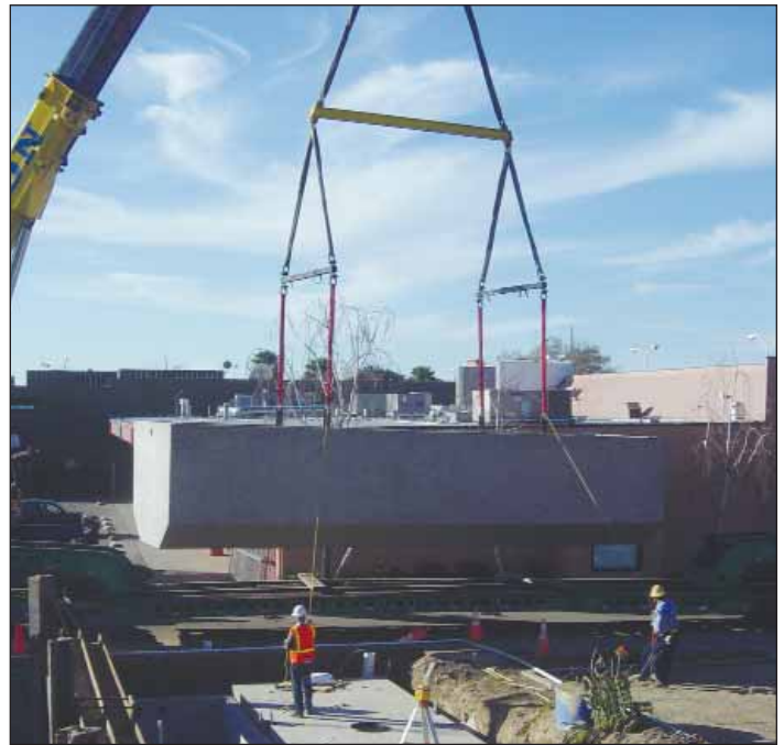
Large concrete tanks required special transport and handling
