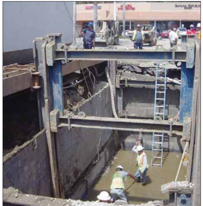
The Double Whammy – Box shoring and Dewatering required for tank installation
