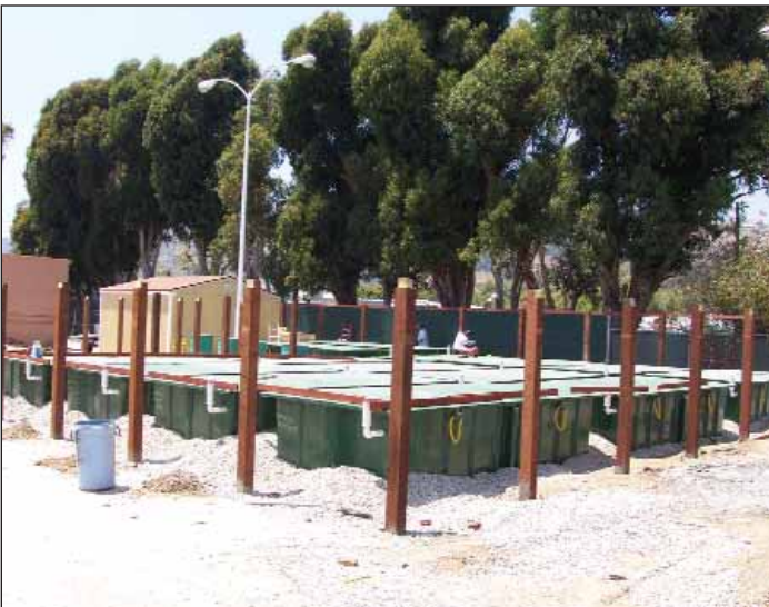
Orenco Advantex Treatment Pods prior to fence installation
