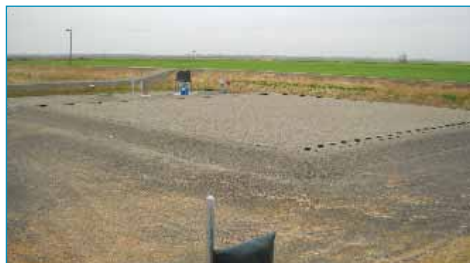
Recirculating Sand Filter
