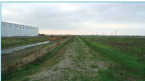
View of construction area before installation of treatment system
