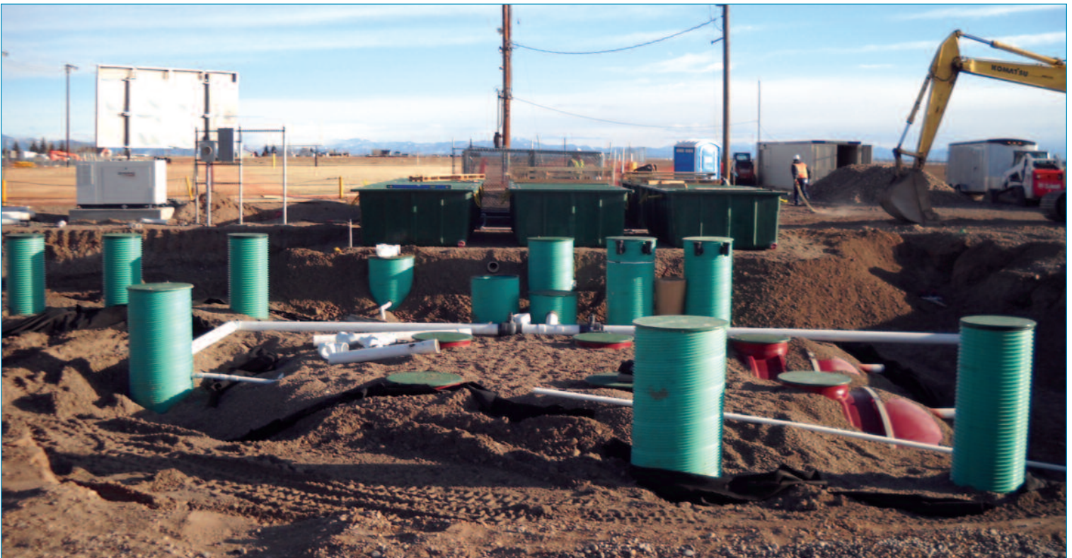
Treatment system being installed
