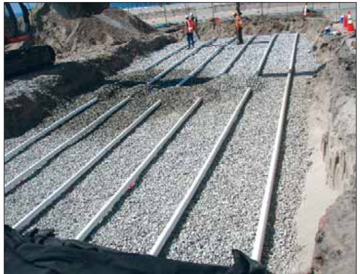
IWS drainfield installation at Zuma Beach
