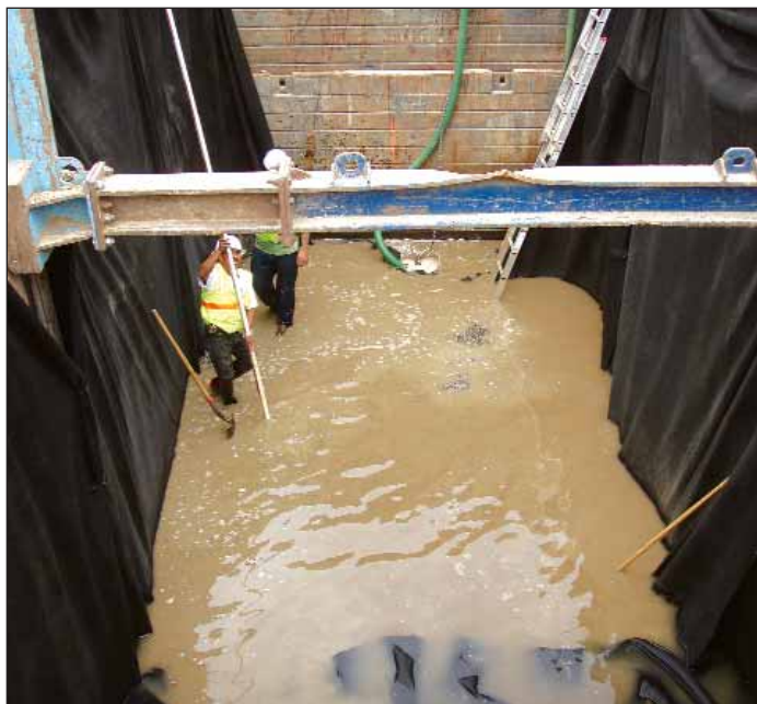
IWS shoring and dewatering of excavation to install tanks
