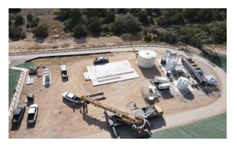
By rapidly deploying BluBox Modular MBR Systems, IWS and MIMBR successfully provided the vital wastewater infrastructure needed to prevent a major housing bottleneck. This phased approach delivered exceptional speed: Phase I in just 44 days, and the Phase II expansion in only five months. In total, this implementation successfully provided the required 150,000 GPD of reuse-quality water, ensuring the essential services kept pace with the community's rapid development.
